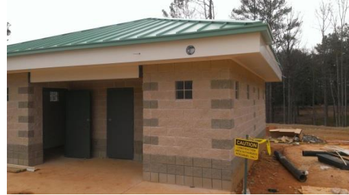
Playground restroom building – Interior work continues.
