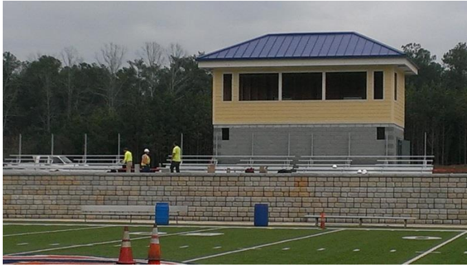
Football Pressbox & Storage Building, bleacher installation.
