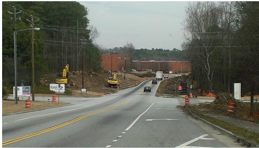
Oakley Industrial Boulevard looking north. Stalwart Drive to the left (Clearing)
