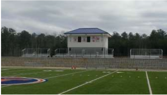
Football Pressbox & Storage Building, bleacher installation.
