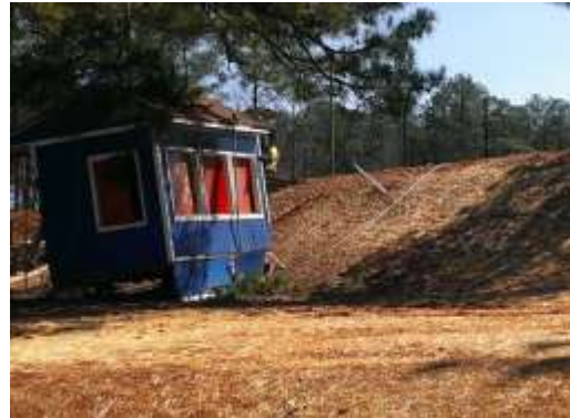
Old pressbox being removed.
