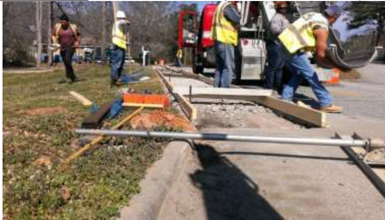
Work crew begins pouring sidewalk at the beginning of March.
