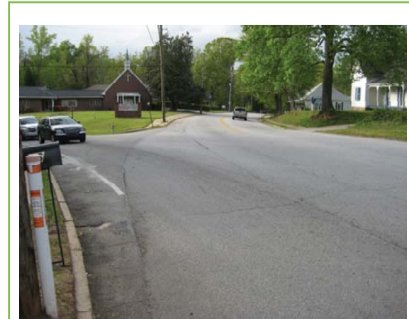
W Campbellton Street at Rivertown Road
