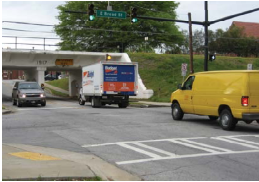
Low bridge on E Campbellton Street
