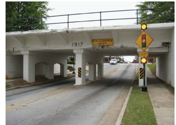
Campbellton Street Underpass
