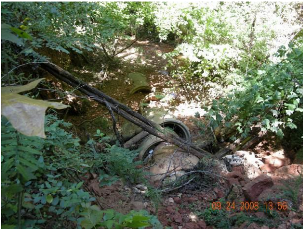
Figure 9: Failing Culvert
