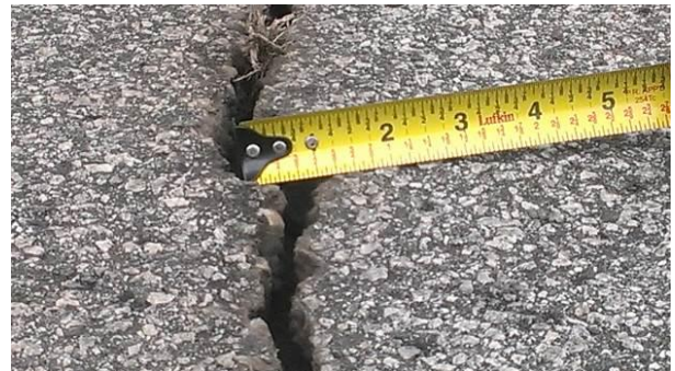
Figure 12: Cracked Pavement
