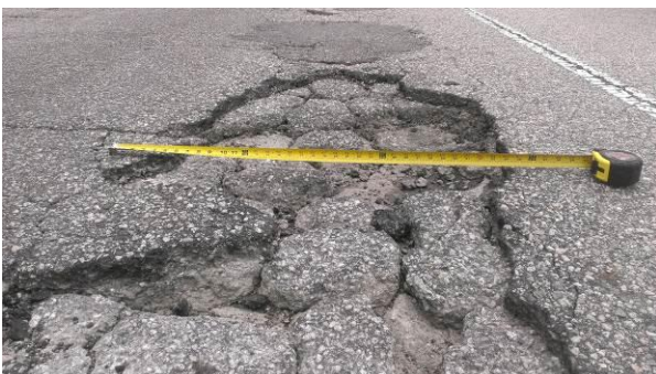
Figure 11: Potholes
