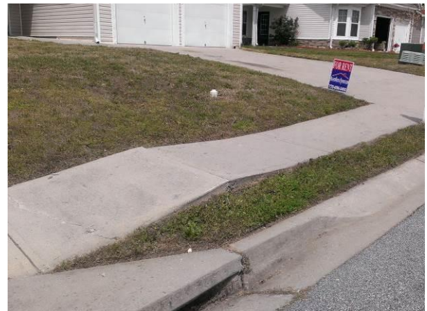
Figure 10: Sidewalk Buckling
