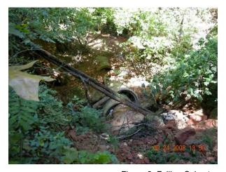
Figure 9: Failing Culvert
