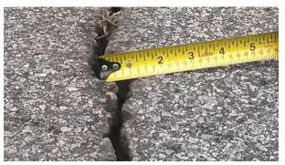
Figure 12: Cracked Pavement
