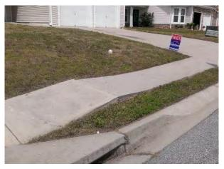
Figure 10: Sidewalk Buckling
