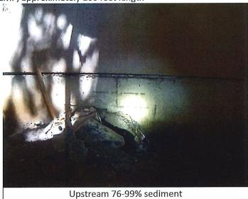
EOP-11061: End of Pipe (downstream of SDPIPE-11062) buried by debris, needs cleaning
