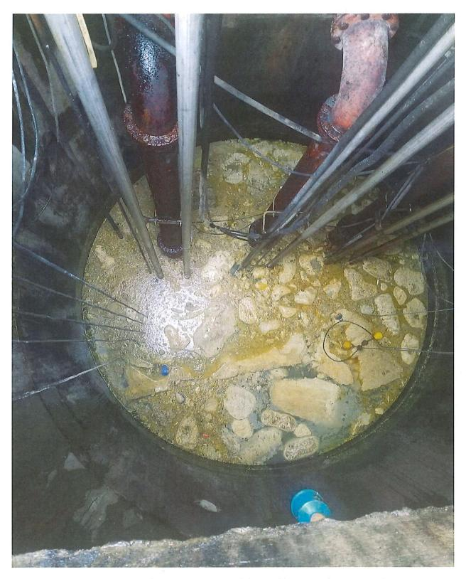
Pump Station full of sewage, grease, and disposable materials. Not pumping.
