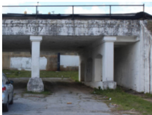
Redeveloped underpass along SE Broad Street.
