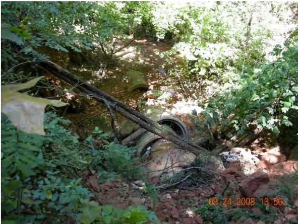
Figure 9: Failing Culvert
