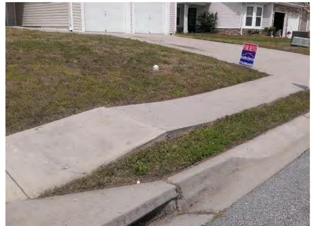
Figure 10: Sidewalk Buckling
